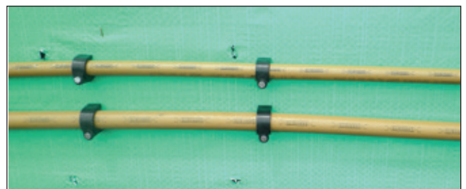
Fig. 3.2 – Installed piping services prior to the installation of Hebel PowerPanel 50
